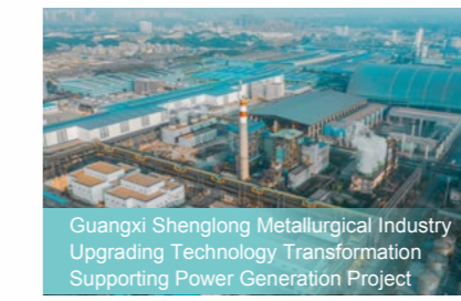
Jiujiang Iron and Steel 125MW ultra-high-temperature subcritical power generation project
