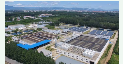
The wastewater treatment plant project in Liangxiang, Beijing
