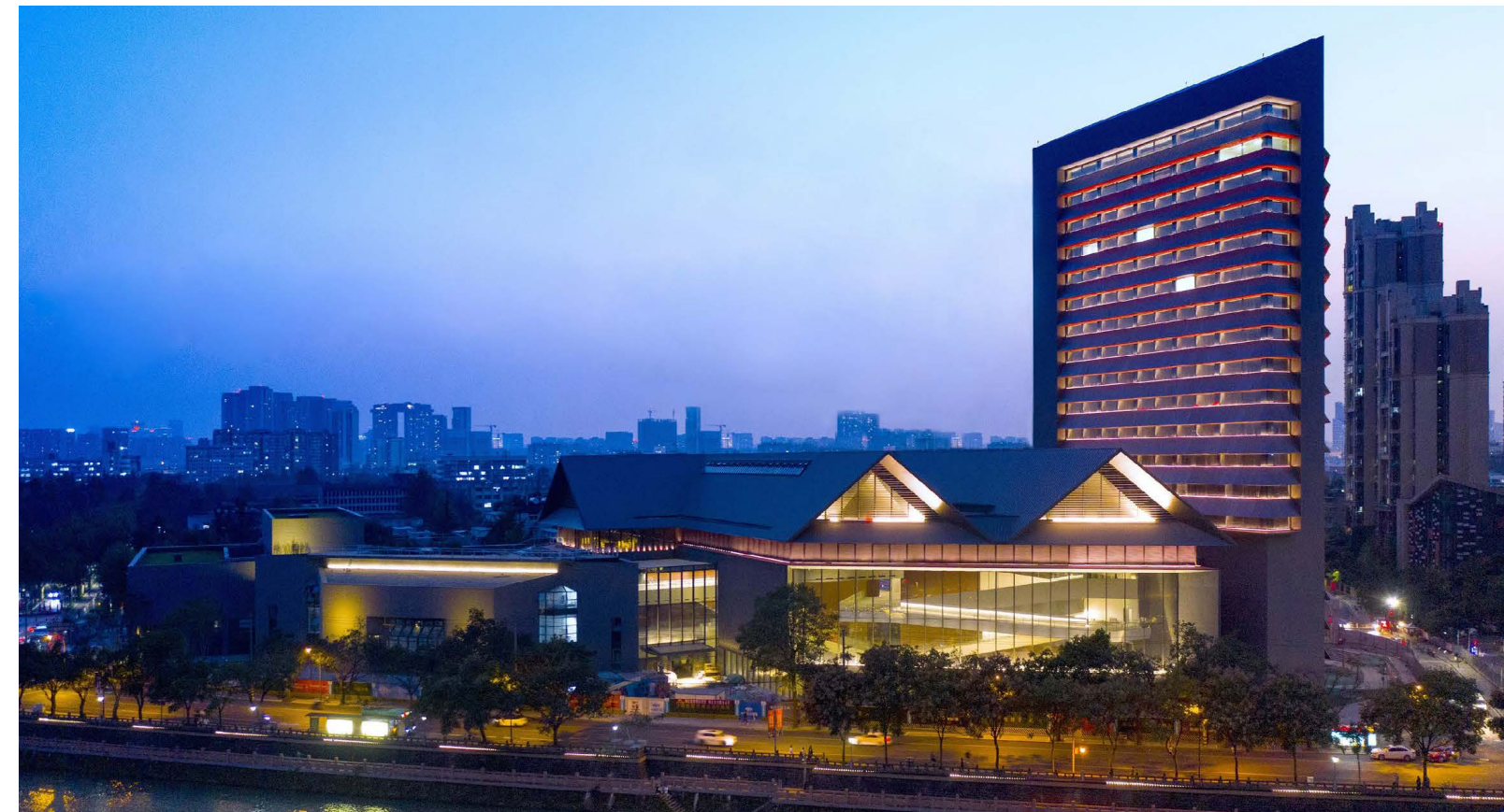
Sichuan University Museum Complex Project
