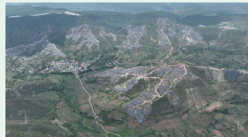
The Taoyuan Photovoltaic Power Station project in Lufeng
