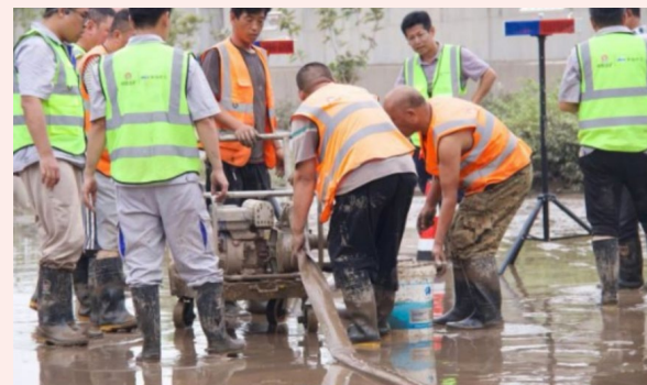
Emergency repair of the sewage pump
