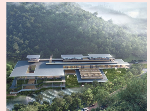
Rural revitalization project in Shaolu Village, Motianling Demonstration Area, Wushan County, Chongqing Autonomous City
